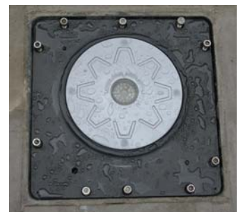
Fig. n: attachment of bollard to frame
