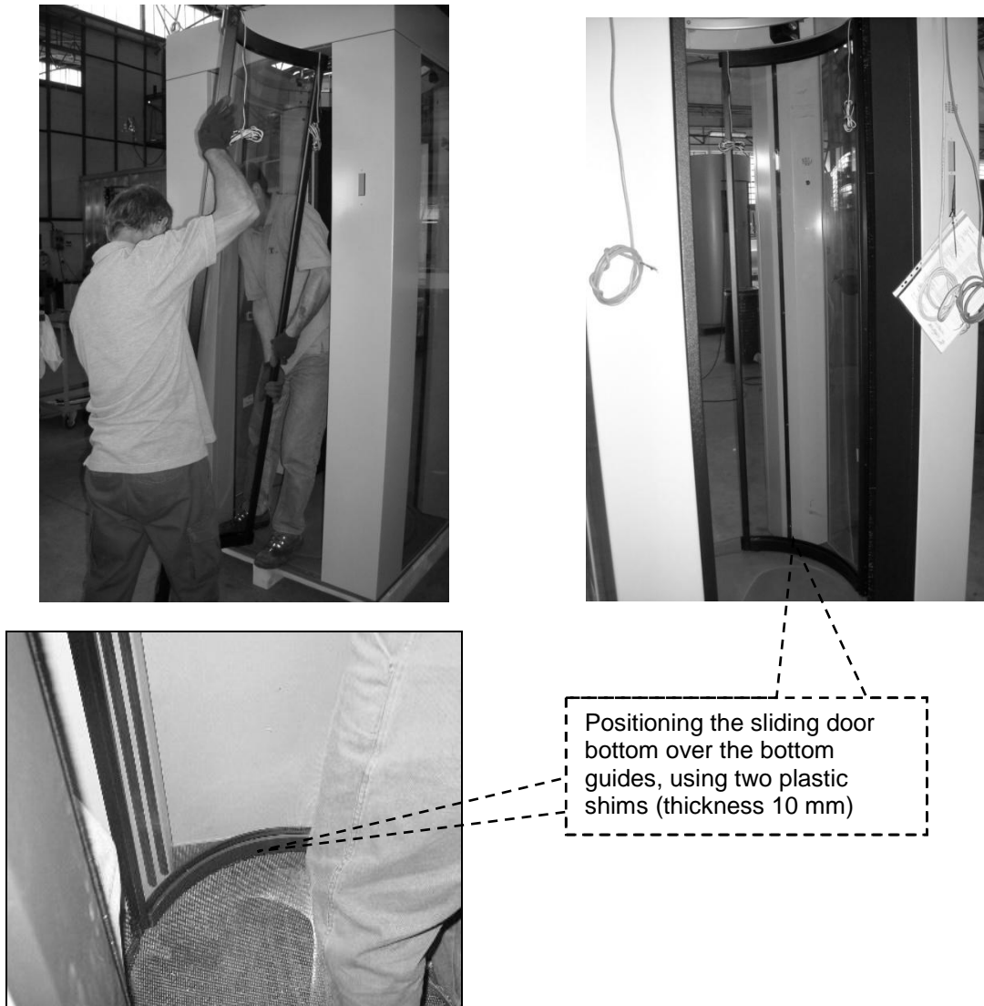
Figure 2-14 Sliding doors positioning inside the booth
